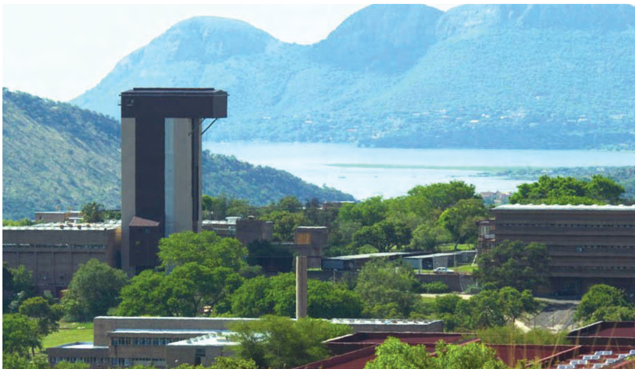
The Pelindaba site of the Helium Test Facility, with the Hartebeespoort Dam in the background. The 43-meter-high facility was built to test the helium blower, valves, heaters, coolers, recuperator, and other components at pressures up to 95 bar and 1,200°C
