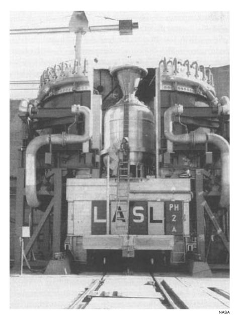
The Phoebus-2A, one of twenty nuclear thermal rockets tested under the ROVER and NERVA programs.
