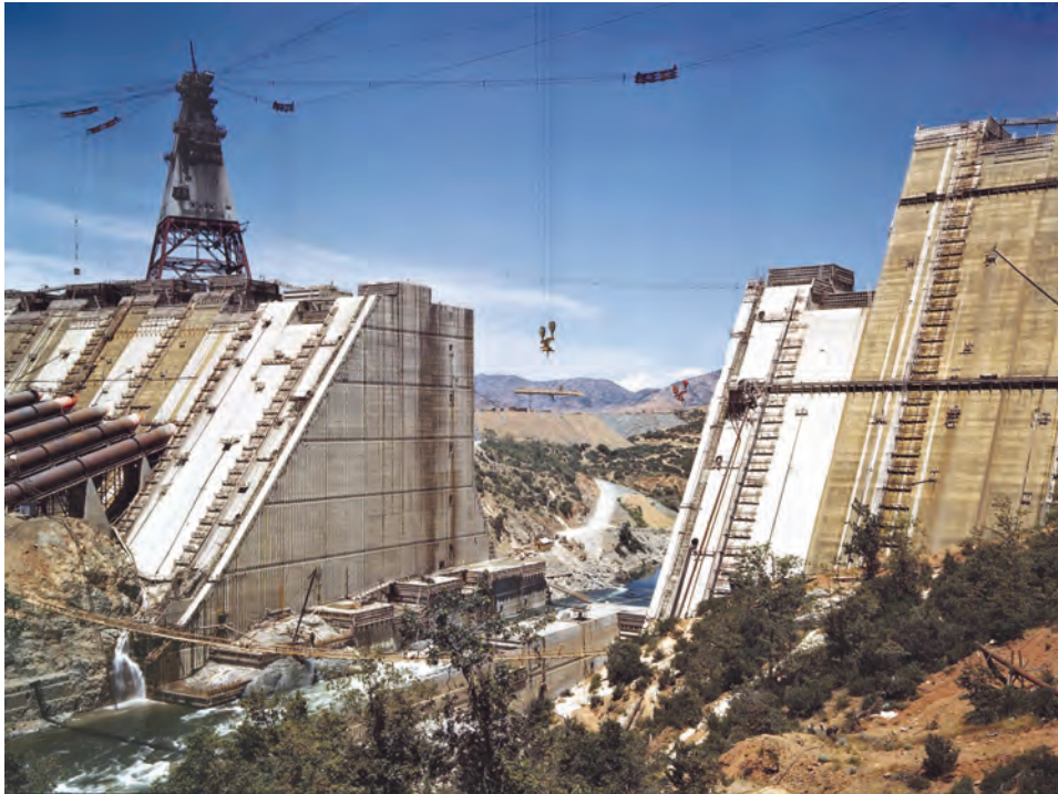
Shasta Dam under construction, June 1942.
