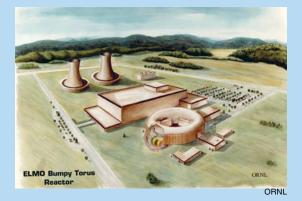
An artist's drawing of an Elmo Bumpy Torus fusion power plant. The EBT uses steady-state electron cyclotron resonance heating to produce a steady-state plasma in a current-free geometry. The design features a hybrid magnetic trap formed by a series of toroidally connected simple mirrors. Operated at Oak Ridge National Laboratory in the early 1980s, the EBT's electron confinement agreed with theoretical predictions. The program was abandoned in 1985.
