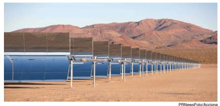
There is no ``free energy'': Here, Acciona's Nevada Solar One concentrating solar power plant, the world's largest, produces less than 15 megawatts of power, averaged over the course of a day.
