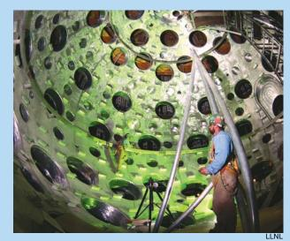
Construction workers install equipment inside the 10-meter diameter target chamber at the National Ignition Facility. The spherical chamber, 10 meters in diameter, is constructed of aluminum panels covered in concrete that has been injected with boron to absorb neutrons from the fusion reaction. The holes in the target chamber permit the laser beams to enter the chamber and provide viewing ports for all of the diagnostics.
