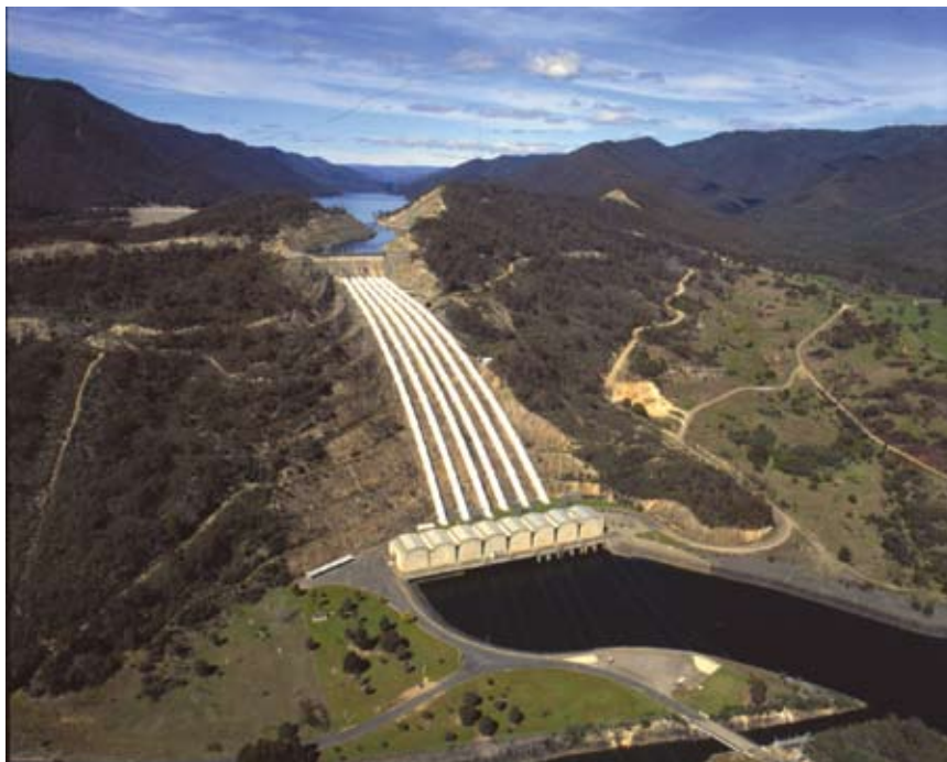
▲ Six generators at Tumut 3 power station. Two of them can provide enough electricity to power a city the size of Australia's capital, Canberra.
