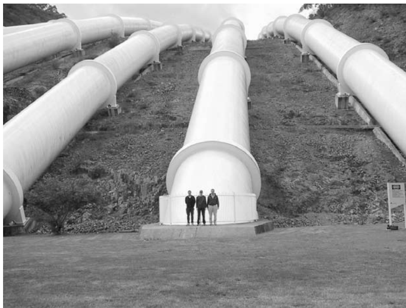
The six pipes ► of the power station Tumut 3 are each 487 meters long, 5.6 meters in diameter, and collectively contain 10,260 tons of steel.
