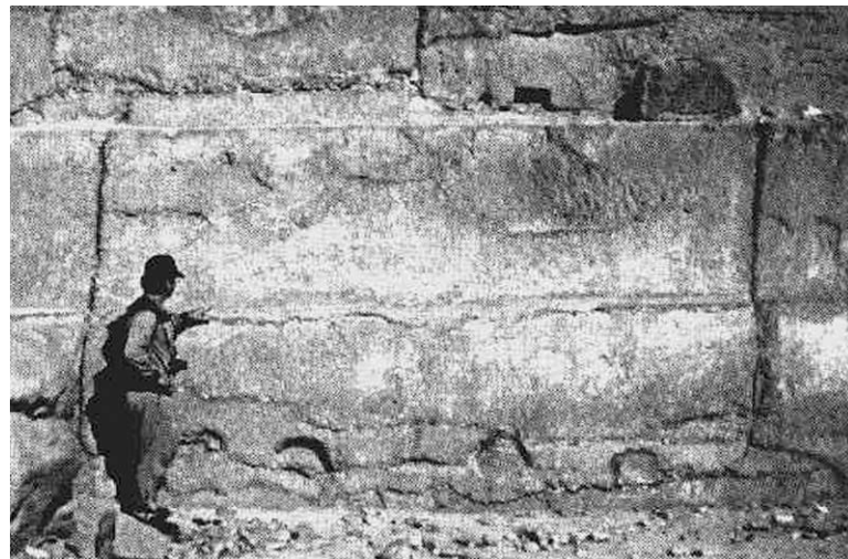
Figure 2 PYRAMID BLOCKS SHOWING CURVED JOINTING
